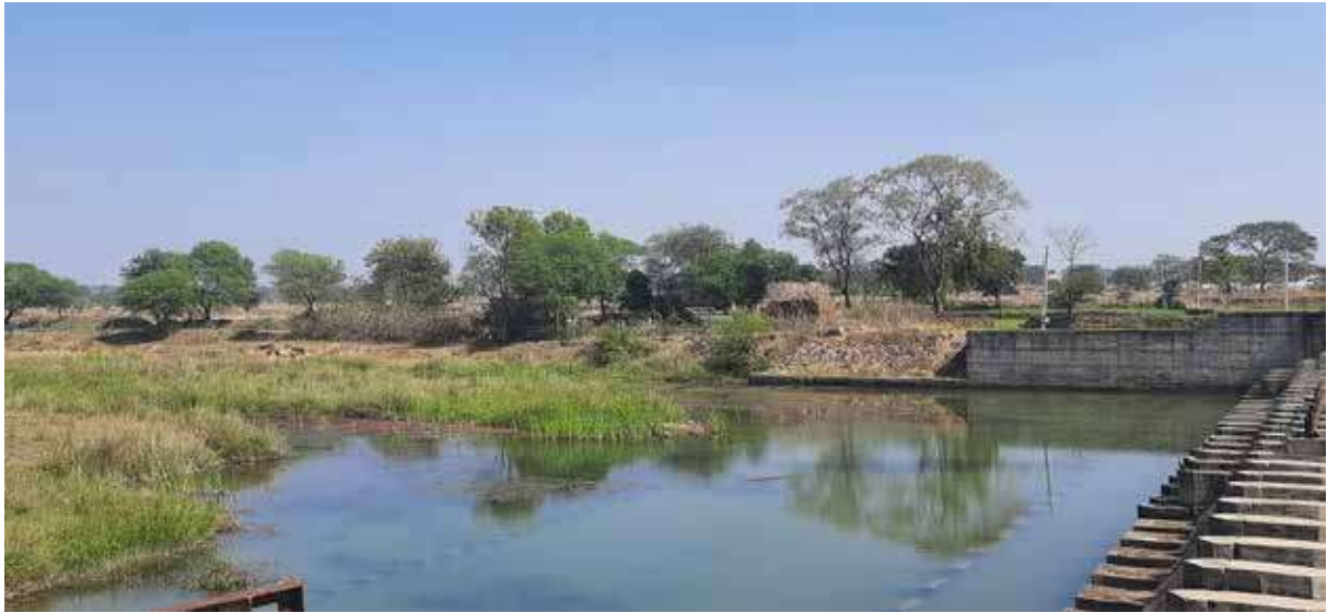
Picture 1 Water harvesting structure, that is, check dam constructed across a stream of Jonk River in Nuapada district
