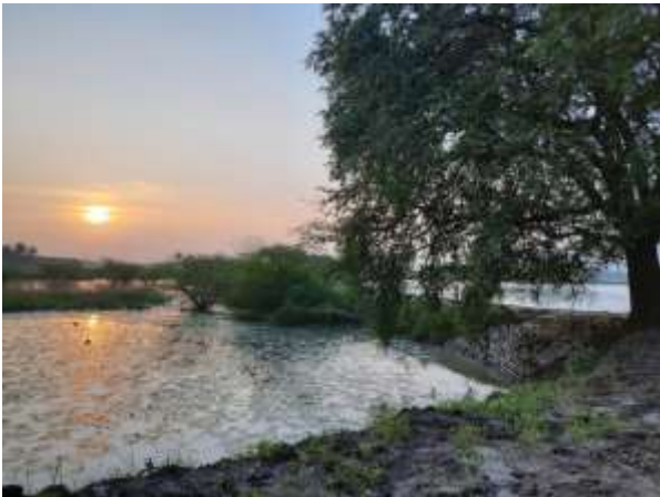
FIGURE 12 Two irrigation tanks separated by a bund in Puducherry region. The silt excavated from the tanks is used for the repair and strengthening of the bunds and also transported to external sites that require silt for construction purposes.
